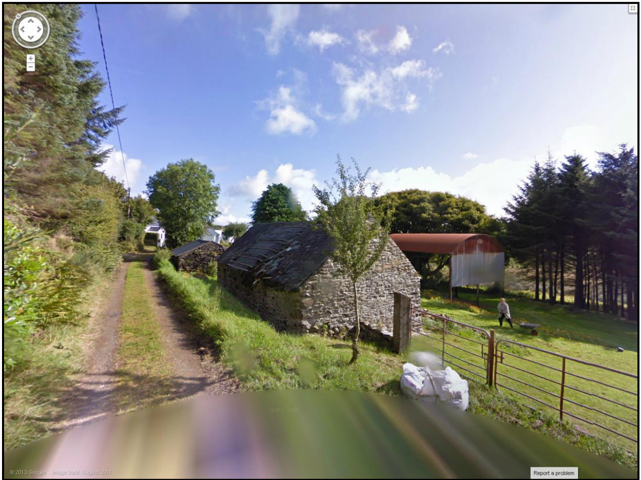
Looking north down the road at some of the buildings of Prison
