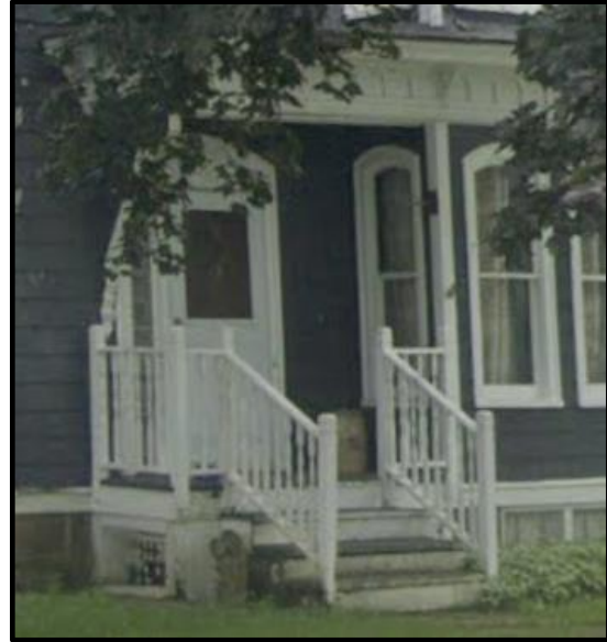
August - 2023. House at the approximate location of the O'Donnell rent house. 3749 Prospect Street
